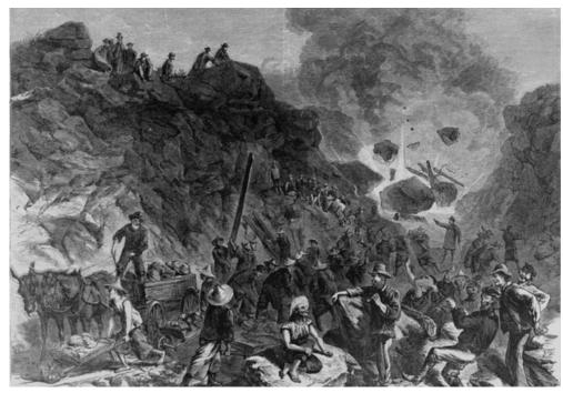
This is a drawing depicting railroad workers removing large rocks in order to clear a path for the railroad to be built. Railroad workers used explosives, as seen in the back of the drawing, in order to break up natural rock formations. This was a very dangerous way of clearing the land for the railroad. This drawing was published in 1869, as the Transcontinental Railroad was being completed.
